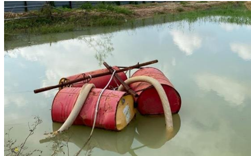
Recycle drum used for ECM water pump for protect from mud
