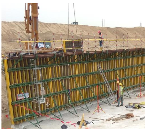
Use of system formwork to reduce timber usage
