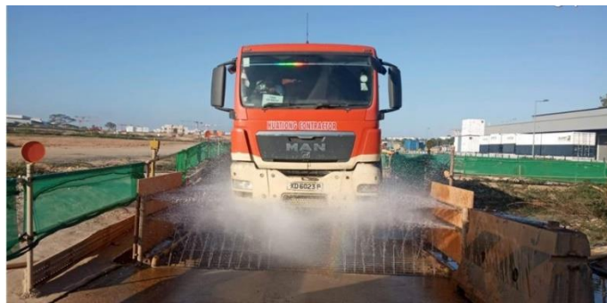
Recycle water from ECM used for wheel washing bay
