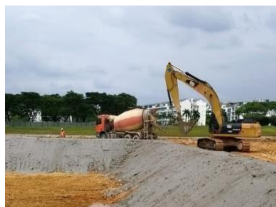
Use of sustainable material LSS for slope protection
