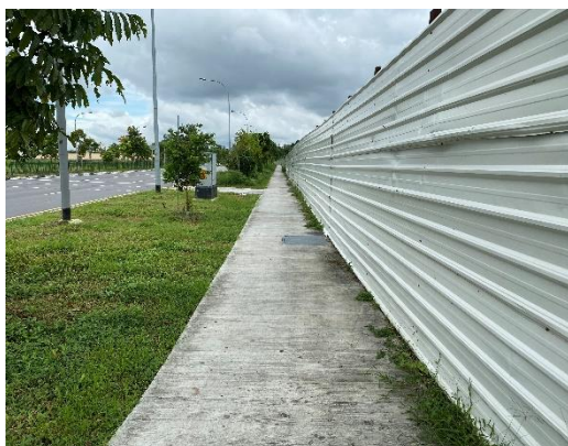
Provided zinc sheet hoarding
